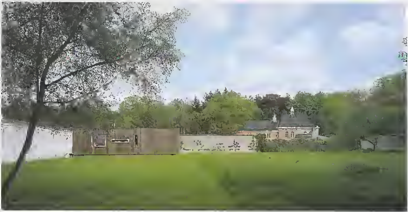
Detalle de extremo Norte de fachada Este / Detail of Northern end, East facade
